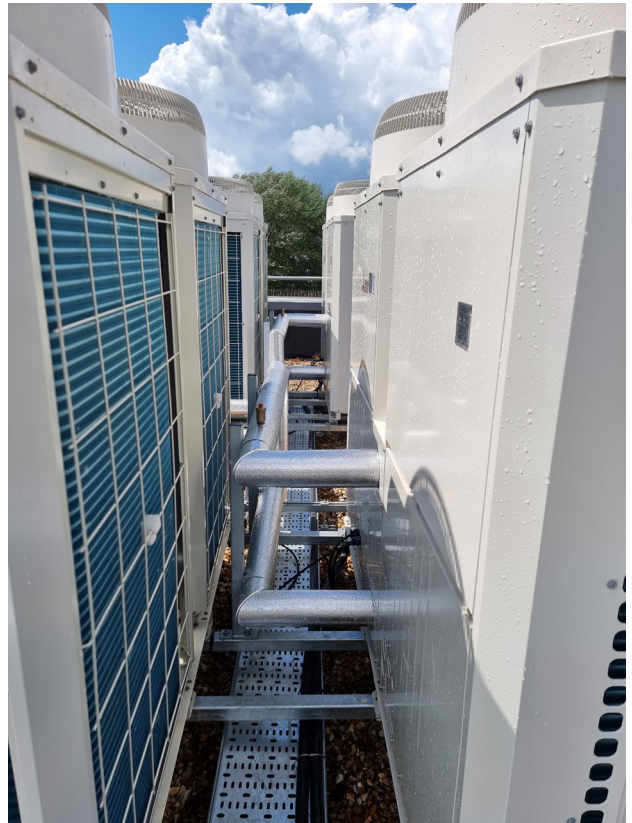
An air source heat pump condenser at City Depot
